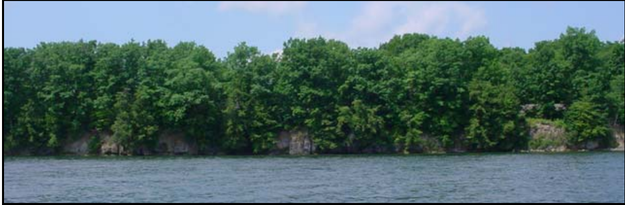
Figure 4.8: A portion of undeveloped lakeshore in the Town. There is not enough space between the railroad tracks and the shoreline in some parts of the Town to allow development along the lakefront. Areas such as this should be retained in their natural condition.
